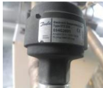
Gambar 4 Expansi Head
