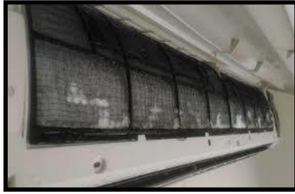
(a) Membuka Filter Indoor
