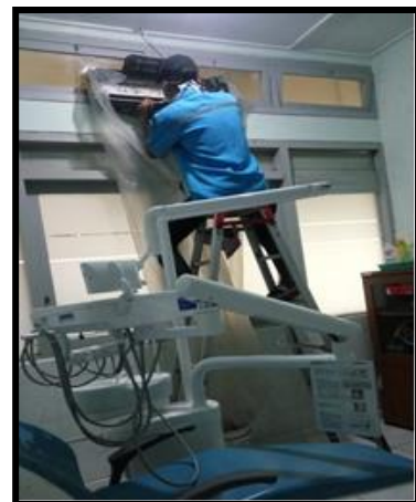
Gambar 4.2 Pencucian Unit Indoor AC
