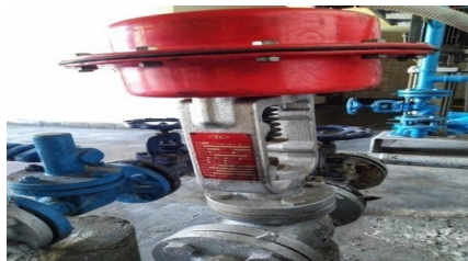
Gambar 3.7 Valve blow down
