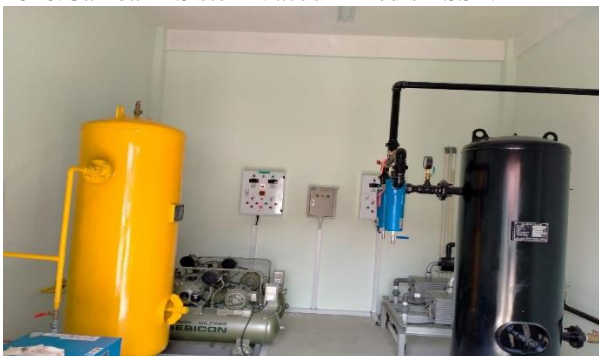
Gambar 1 Sistem Vacuum Medis RSST
