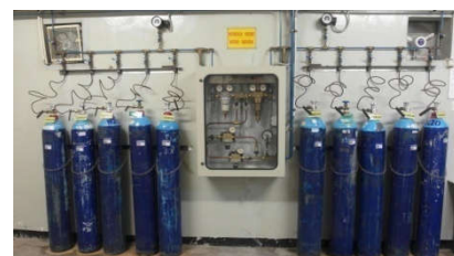
Gambar 3 Sentral Gas Nitrous oxide Tabung
