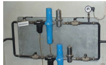
Gambar 7 Filter udara
