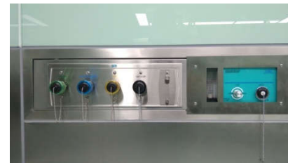
Gambar 12 Outlet gas medis pin indek
