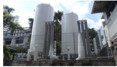
Gambar 1 Tanki liquid Oksigen
